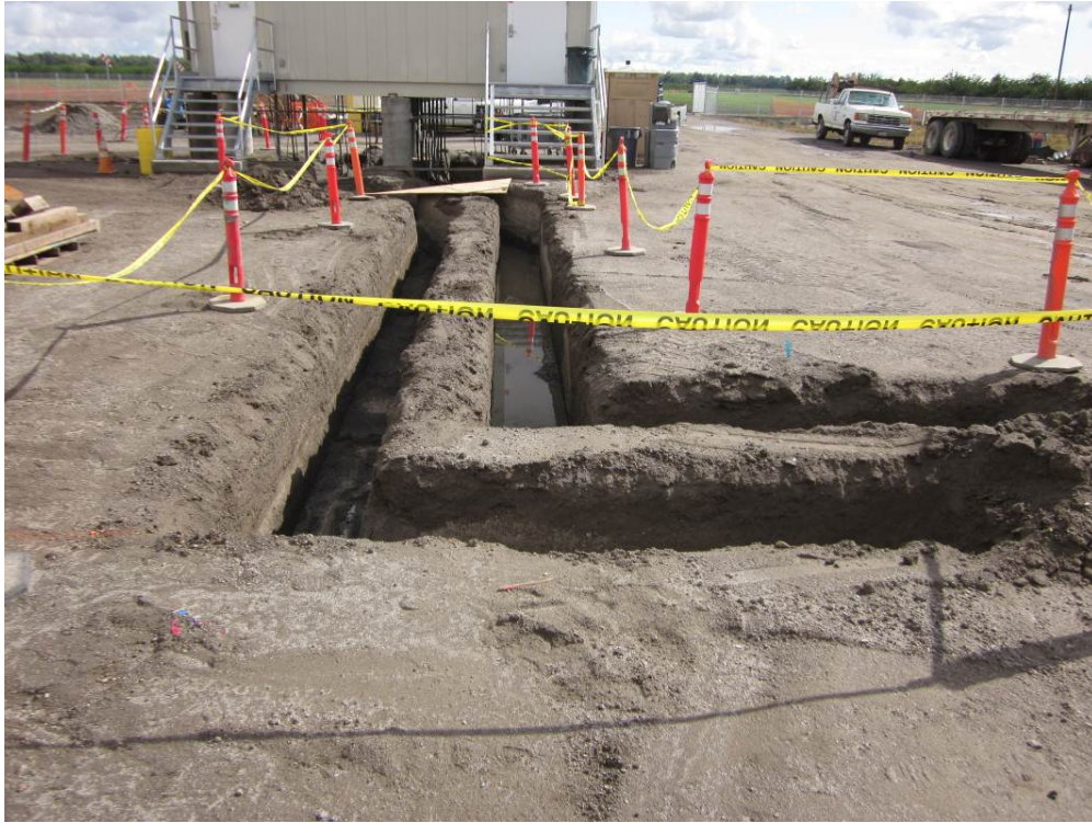
Photo 1: Trenching for buried electrical lines at the Remote Well Pad site.
